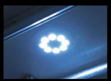
4 recessed flat ceiling lights with 8 LEDs with interior time switch.
